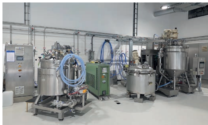
The new production hall
